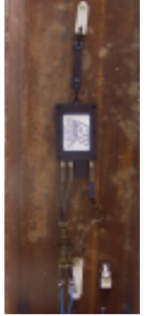
G2's pile driving analysis technology at work
