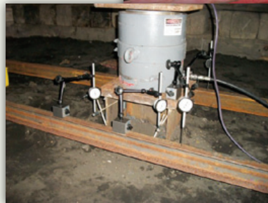
G2 conducts static pile load tests on this foundation. More than 900 piles support the new bridge structure.
